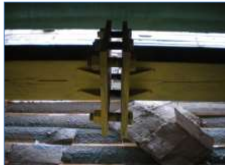
Pre-stressing Mechanism in Truss
