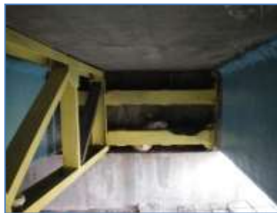
Connection of truss over main beam
