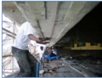
Groove for carbon Fibre composites laminates
